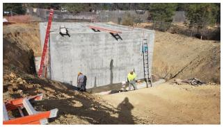
The construction of the Aeromod activated sludge process unit. The Aeromod treatment unit has had all the forms removed and is currently being water tested. Photo by Roy O'Connor.
